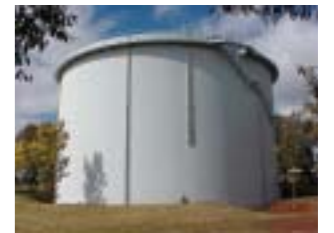
CLEAR WATER STORAGE Total Storage 85.9 ML
