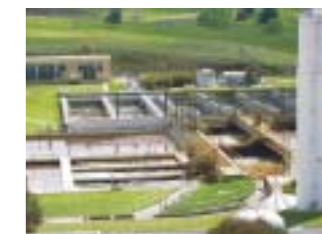
SEWERAGE TREATMENT PLANT
