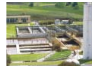
SEWERAGE TREATMENT PLANT
