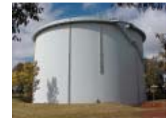
CLEAR WATER STORAGE Total Storage 85.9 ML
